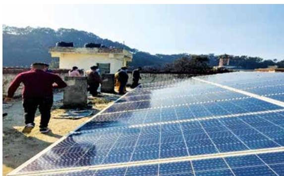
OnGrid Photovoltaic Solar Power plant of 7 kwp
