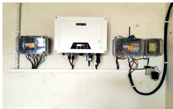
OnGrid Photovoltaic Solar Power plant of 7 kwp
